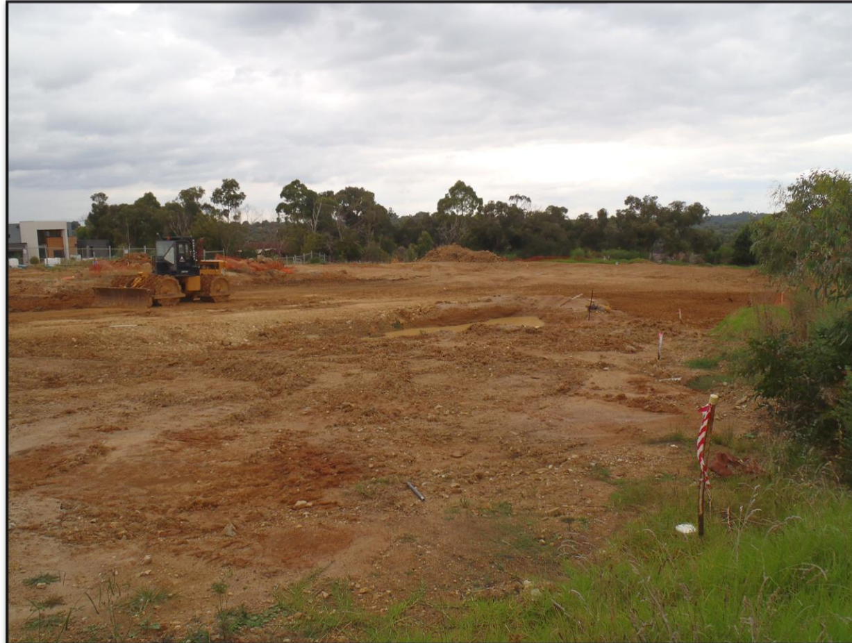
Backfilled Excavation Following Remediation
